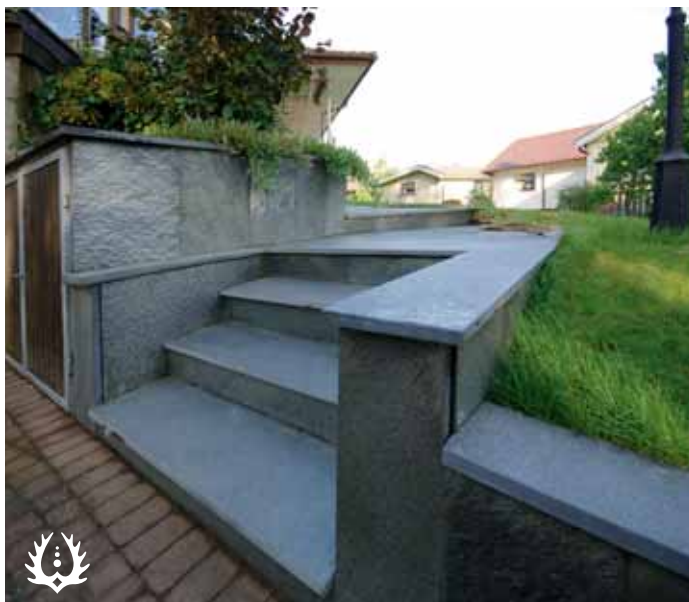
Offerdal Quartzite: Coping and Wall bricks/Dry walls
