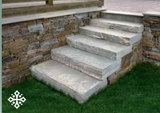
Oppdal Quartzite: Massive treads- natural and sawn edge.
