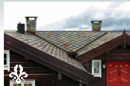
Otta Phyllit: Roofing slates (regular) - snapped edge.
