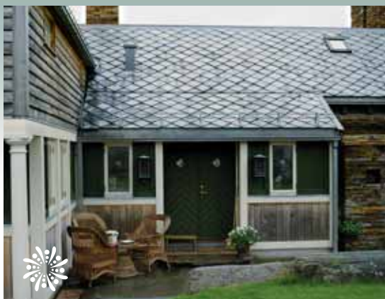
Alta Quartzite: Roofing slates (regular) - snapped edge.
