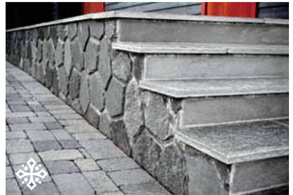
Oppdal Quartzite: Risers and stair treads - natural surface - broken edge.
