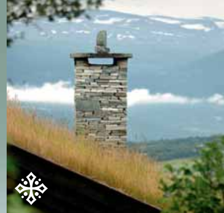
Oppdal Quartzite: Chimney caps and Wall bricks.
