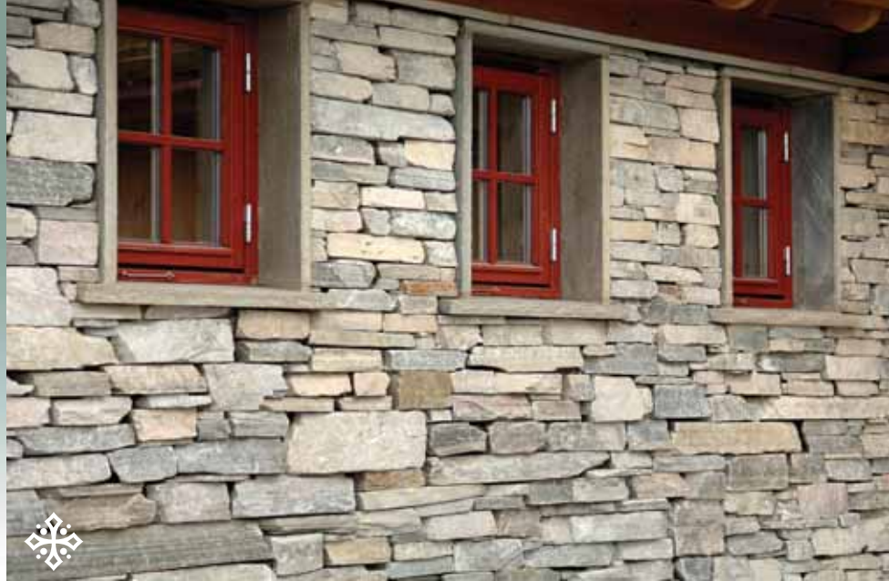
Oppdal Quartzite: Windowsills and wall with Bricks/staved
