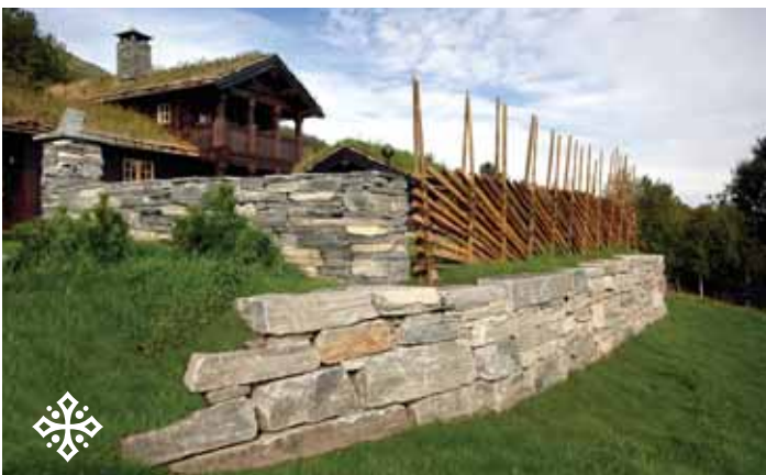
Oppdal Quartzite: Wall bricks / Building blocks.
