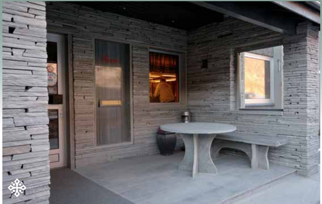
Oppdal Quartzite: Table top, underbody, benches and Wall bricks/ Dry walls - broken edges
