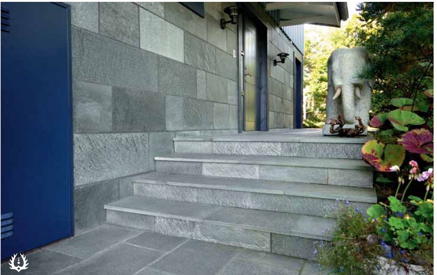
Offerdal Quartzite: Stairs treads and risers - natural riven surface.
