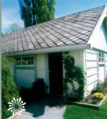
Alta Quartzite: Roofing slates (regular) - snapped edge
