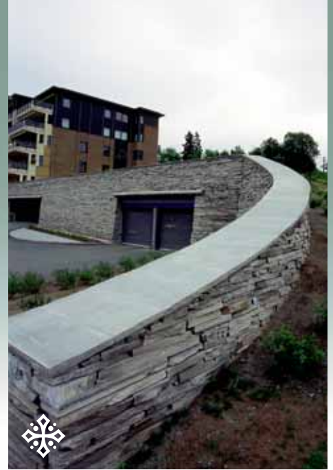
Oppdal Quartzite: Coping and Wall bricks.
