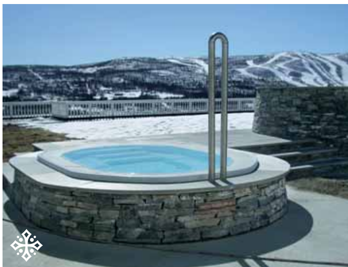
Oppdal Quartzite: Coping and Wall bricks.
