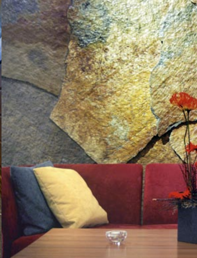
Ottaskifer: Forblending med store bruddheller (overlapp)
